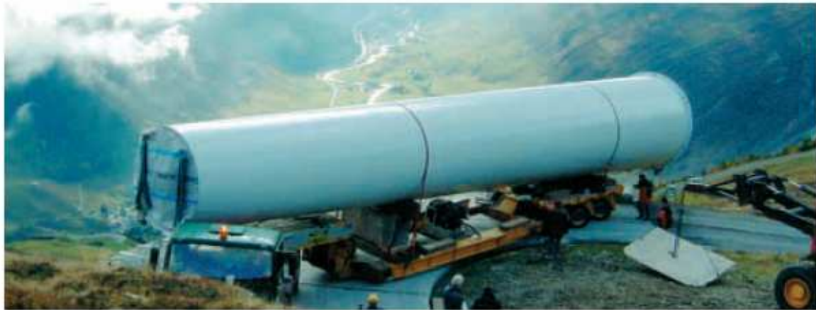
Tricky: The transport of a tower part for an E-40 on the GÜtsch with 2,323 metres height.
